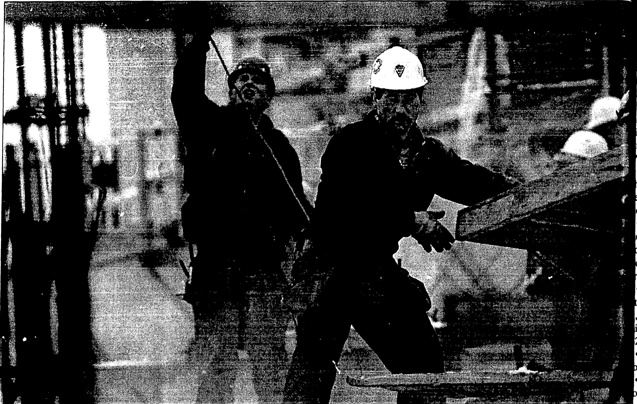
Construction is always booming in Whistler. The best time to apply for a building permit, say municipal staff, is during the
