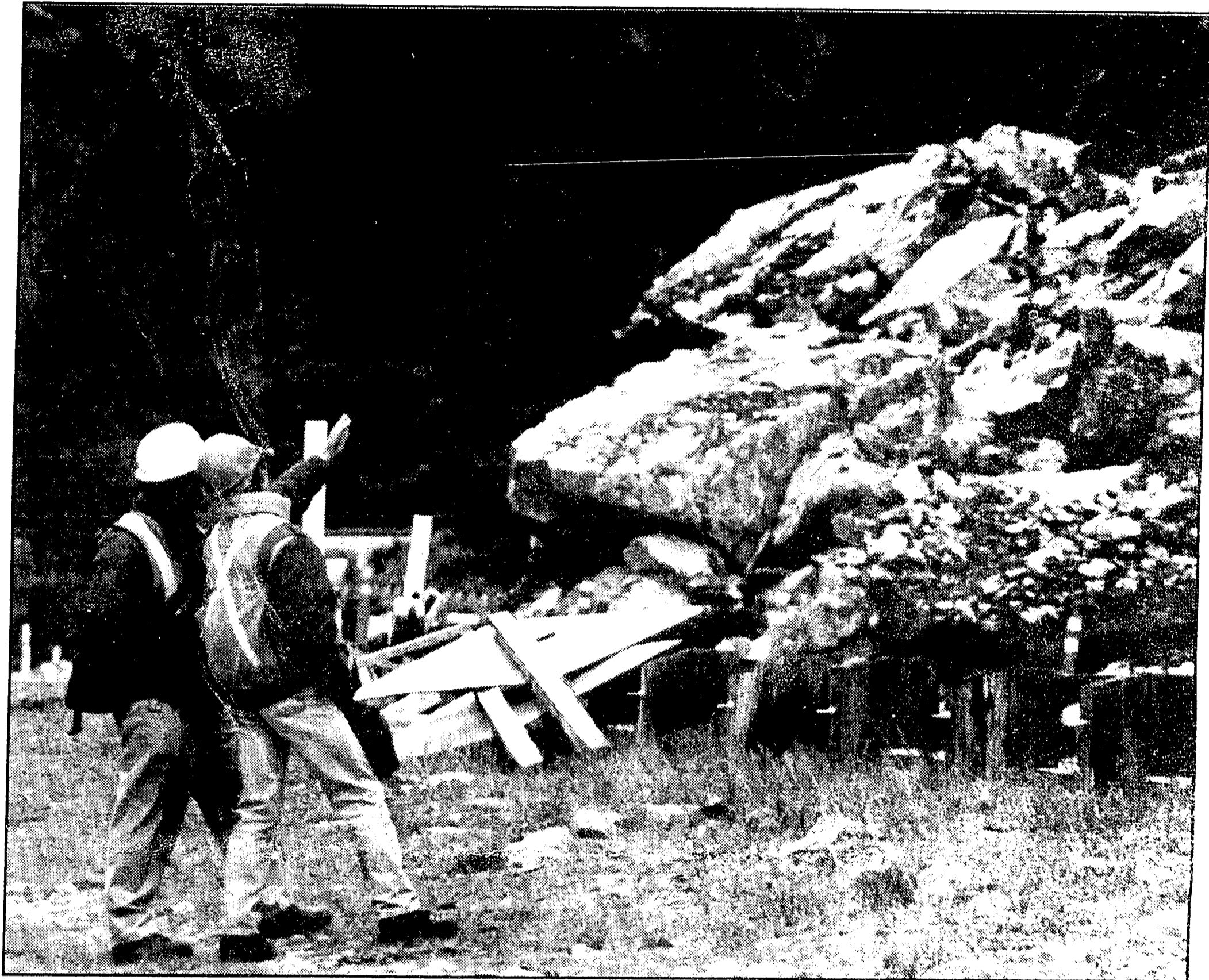
The Ministry of Transportation and Highways continues to monitor the area of recent rockslides in the Cheakamus canyon north of Squamish. Brian Goldstone photo
