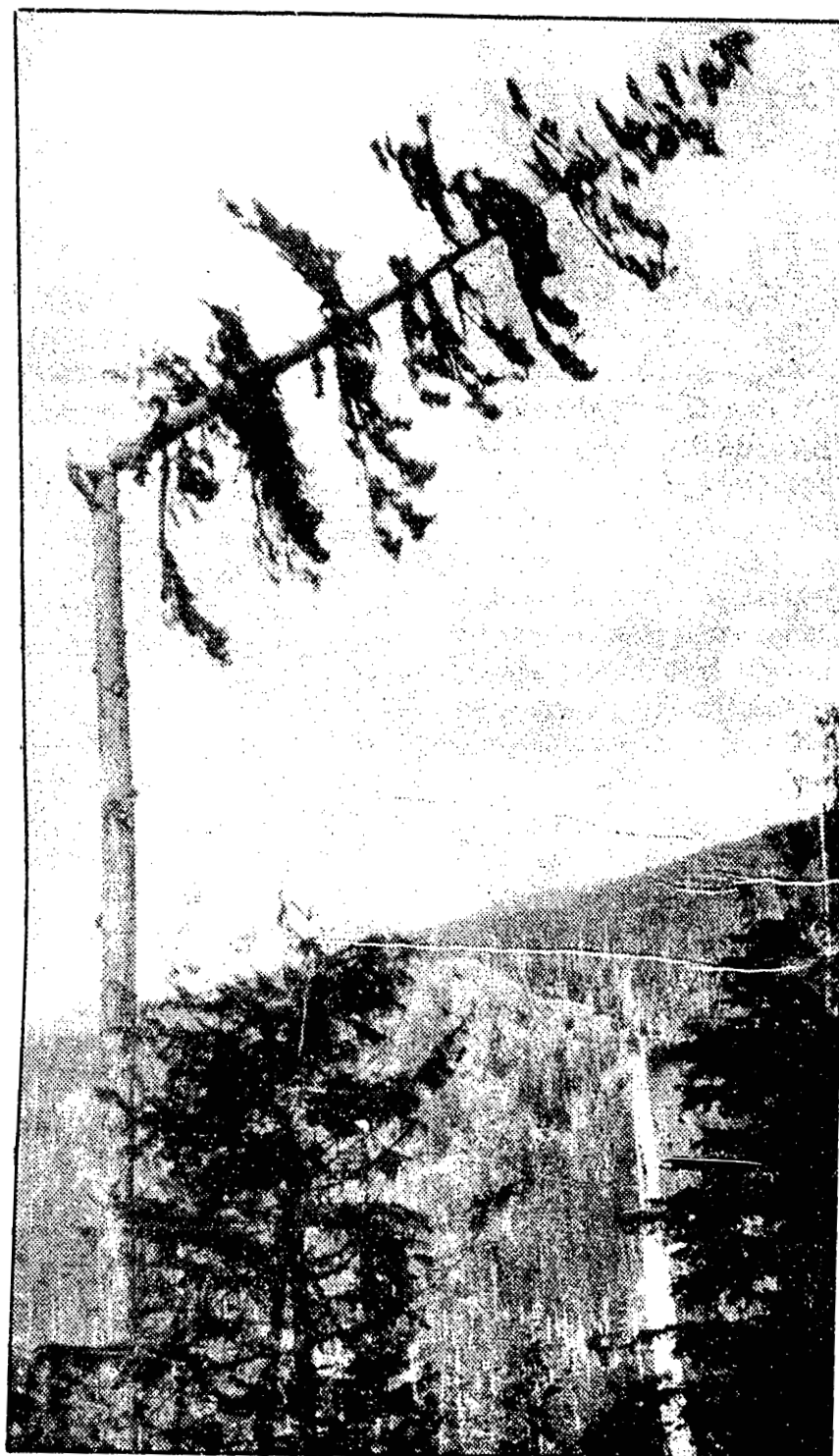
THE REAL THING --Topping a spar tree was all in a day's work back before industry began to use a steel pole for this centrepiece of the woods.
