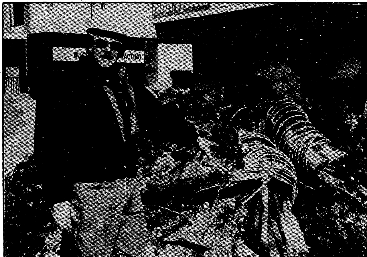
Old wooden culverts unearthed on Cleveland are pointed out by Dennis Cofield.
