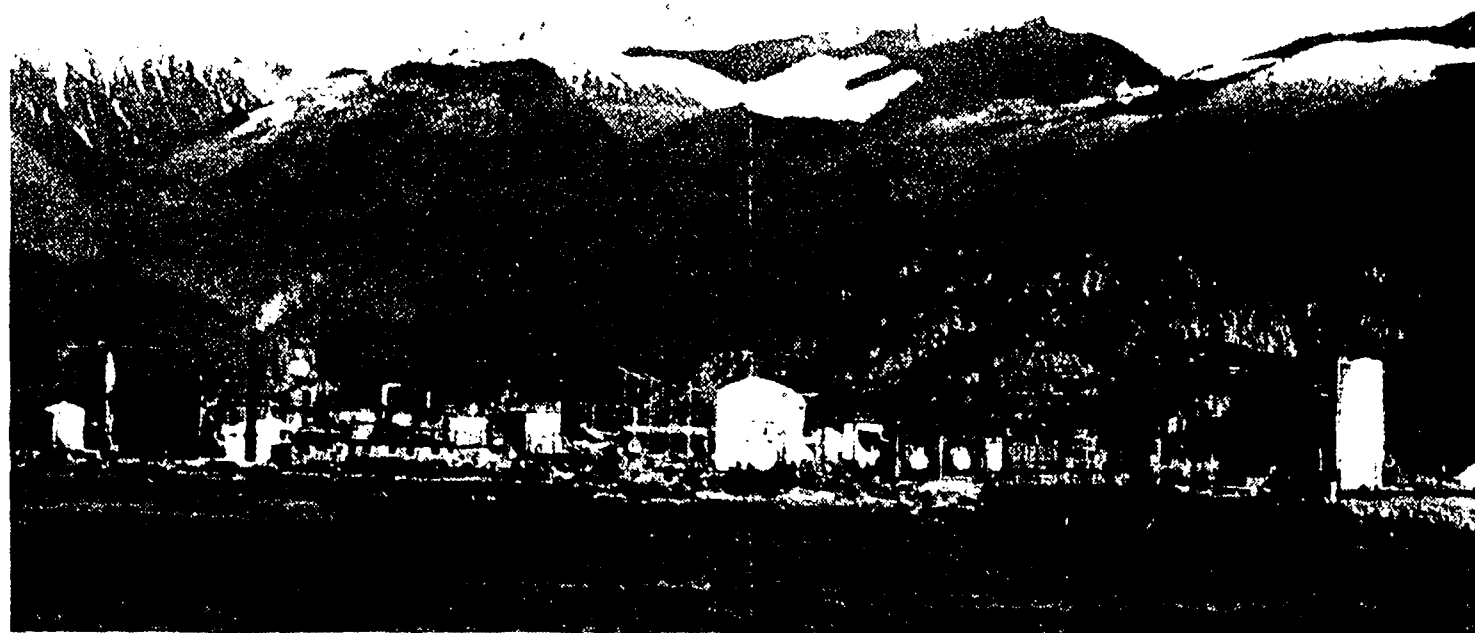
Nestled between Mamquam Blind Channel and Squamish Terminals, FMC of Canada plans an expansion project to produce hydrogen peroxide at the rate of 10,000 tonnes per year.
