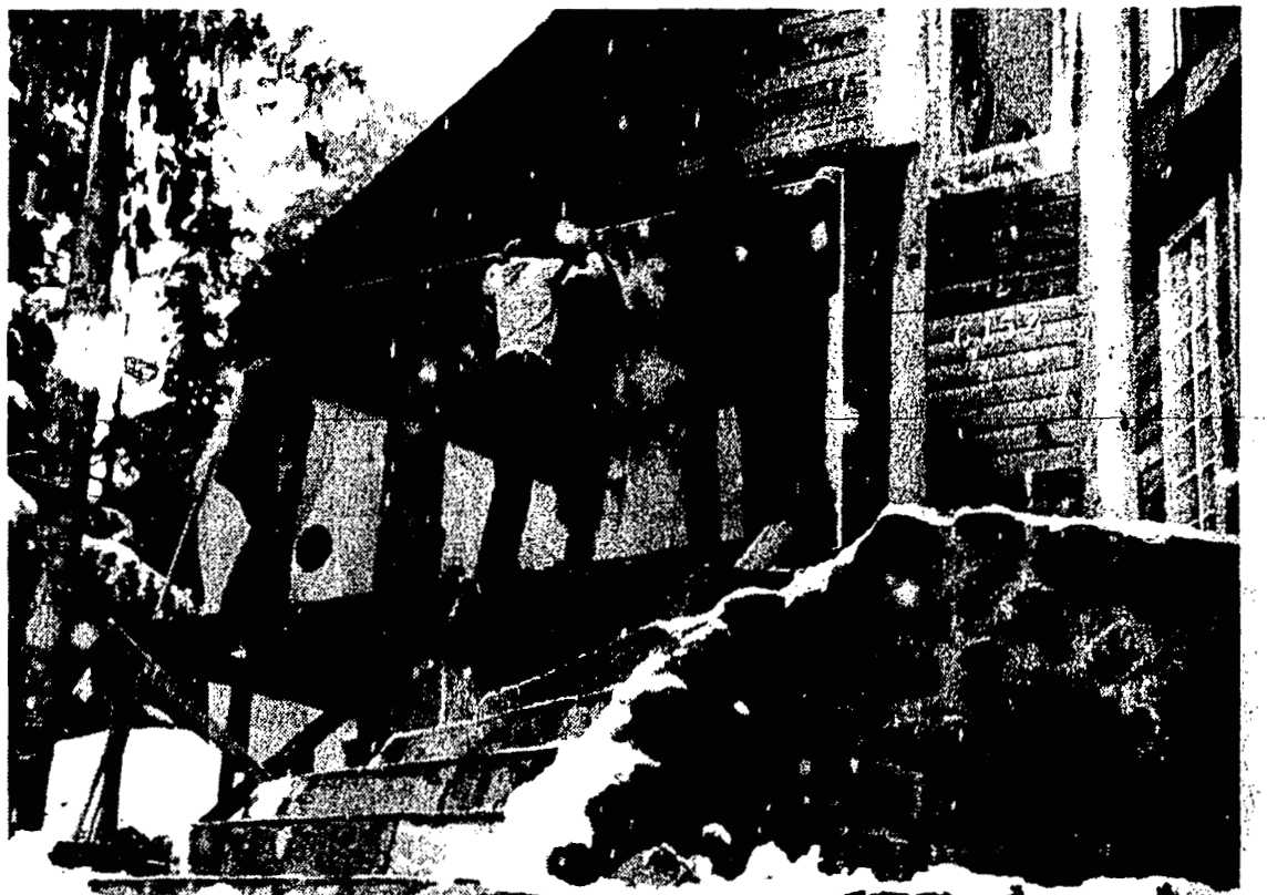
Once the glass unit had been carried up the stairs it was simply a matter of fitting it into the window frame. (Photo by Pete Peterson)
