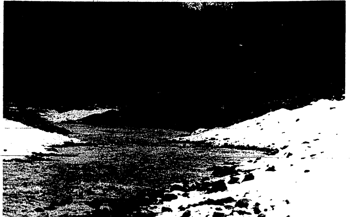
Restoration work has begun on the Stawamus River. It is being returned to its pre-flood condition after it swelled during high waters late in 1981. The work is being done under the emergency program and is expected to be completed by March 15.
