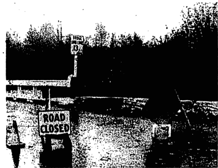
These signs at the south end of the old Mamquam bridge were posted during the height of Saturday's flooding when the trailer court and road were flooded.
