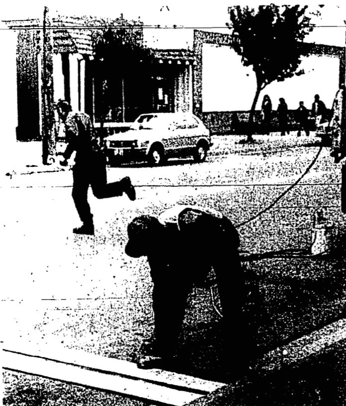
The municipal works crew spent several days painting in parking stall lines on Cleveland Ave.
