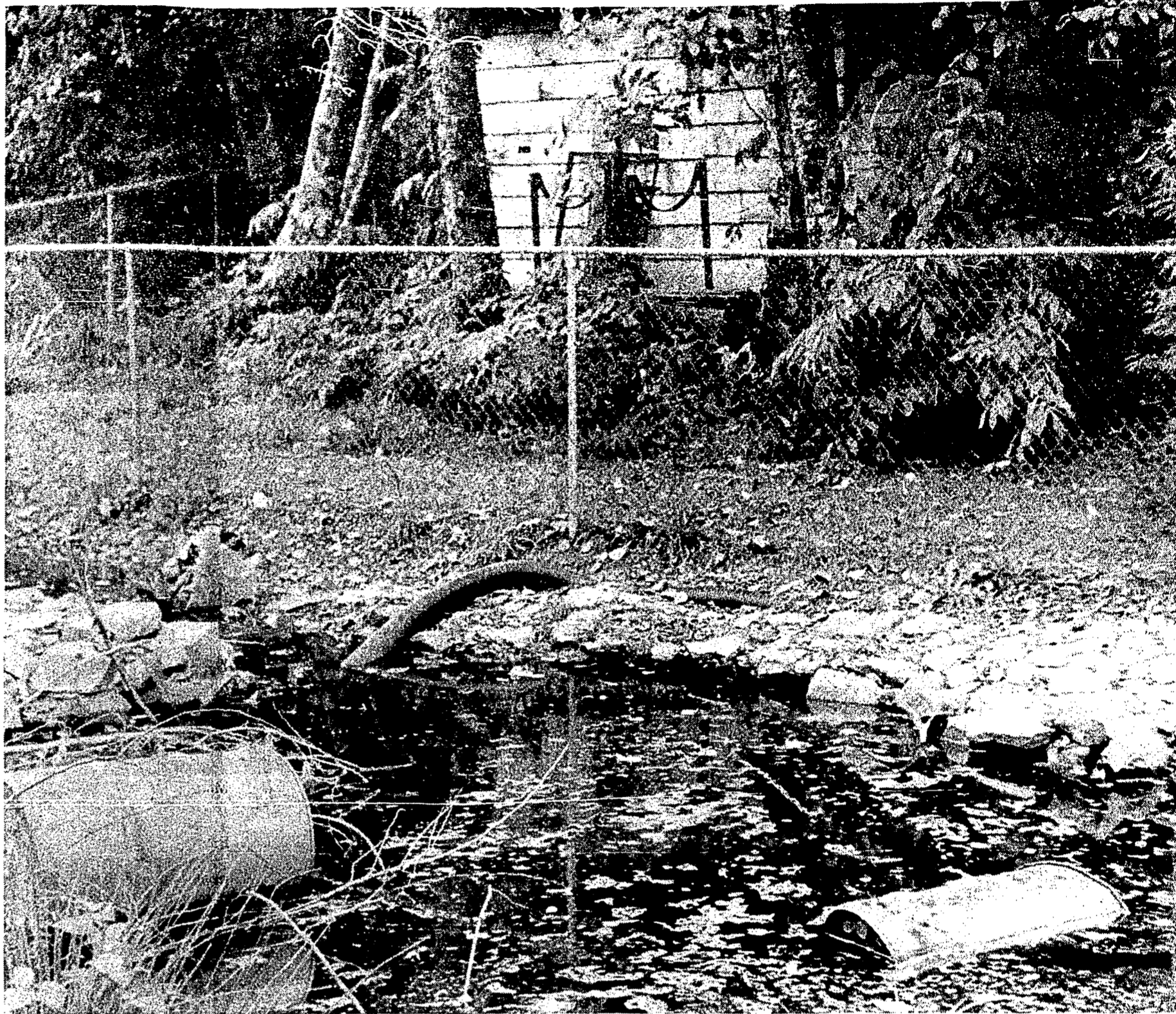
Vandals have kept parks crews busy at Cottonwood Park. Here oil drums lie half submerged in what was at one time a pretty shallow pond. In the background notice the heavy wire fence that neighbours have erected to
