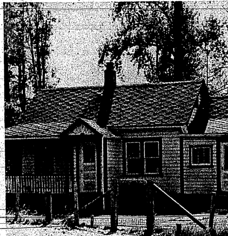
SITTING SNUGLY beside the railway tracks where the golf course road joins the highway is the former Armstrong home. Probably built during the First World War, the location was chosen for its high ground by Bert Armstrong. There he lived with his wife, the former Minnie Rae and his children. After his death his wife lived there until her passing a few years ago. Like the Thorne place just behind it is clearly visible to anyone driving up the road.
