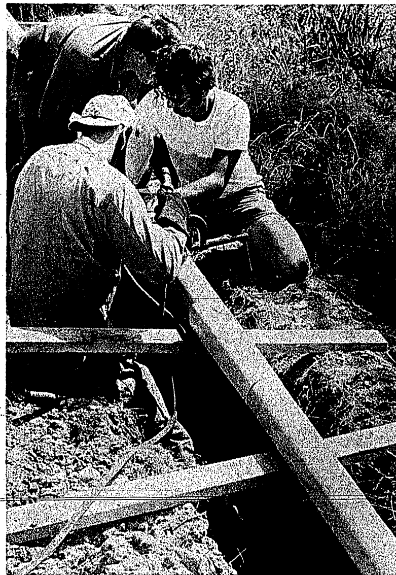
DON KENNEDY, Al Cumskey and Murray Johannsen, putting together a section of the new gas pipelines to Valleycliffe.
