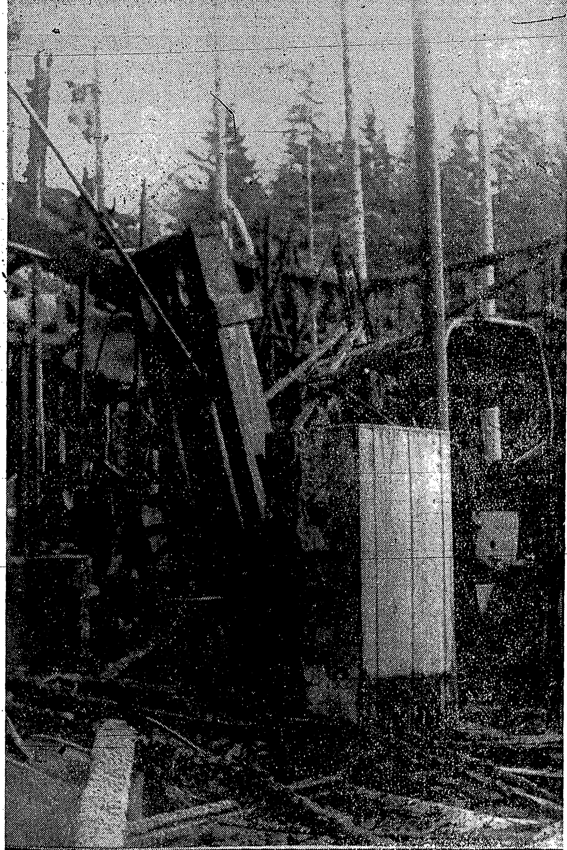
THE CHARRED inside of the garage at Snocap Service after the early morning fire which completely gutted the interior of the building.
