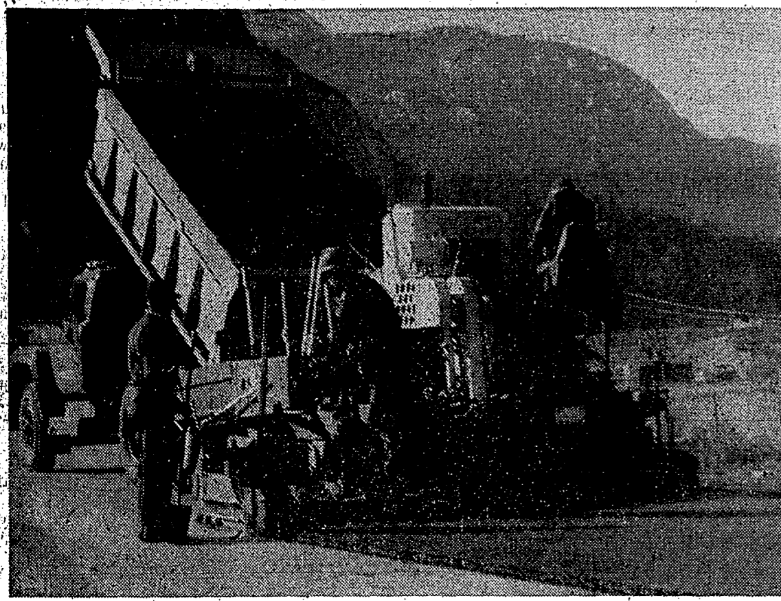
BLACKTOPPING machines were busy putting the finishing touches to the paving of the access roads to the new bridge last week. Work was finally completed late on Saturday
