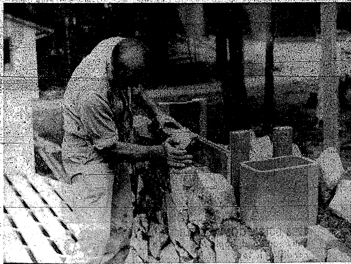
HERE Dick Heinen who is an artist in stone puts the finishing touches on the massive stone chimney of the Bellis home.
