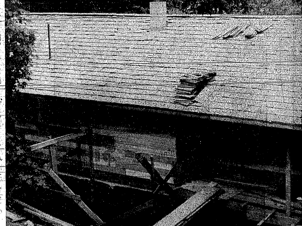
FRONT VIEW of the A. C. Finter home in Garibaldi Highlands. This shows the shake roof and Mrs. Finter says she had the blisters to prove they split the shakes themselves. The Finters are living in the house while they work at completing it. The rear windows overlook the small park and winding stream.
