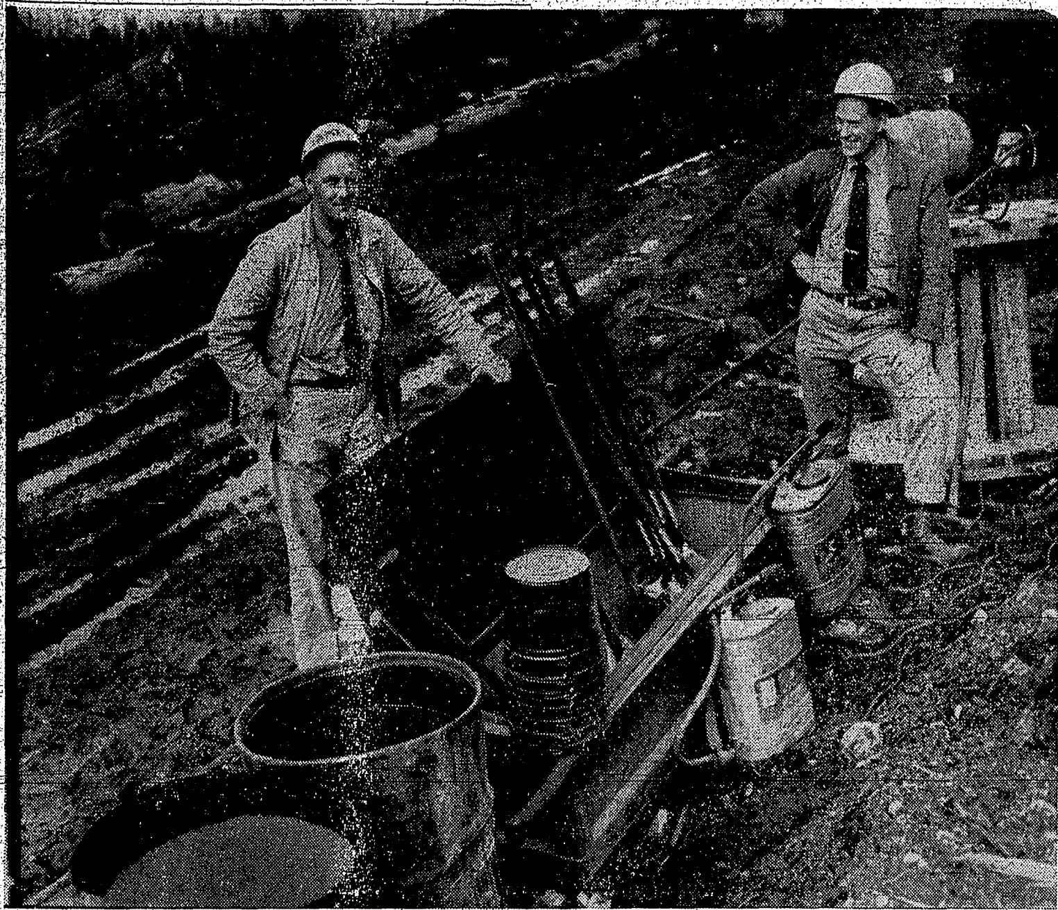
ON LOCATION assistant rangers Jim Price, left, and Don Ferrier inspect tool-box of Van West Logging which includes three axes, three mattocks, six shovels, six buckets, two hand pumps and two barrels of water. One barrel of water is required for each machine, in this case the yarder and loader. If the machines were operating one-half mile apart another and similar box of tools would be needed.
