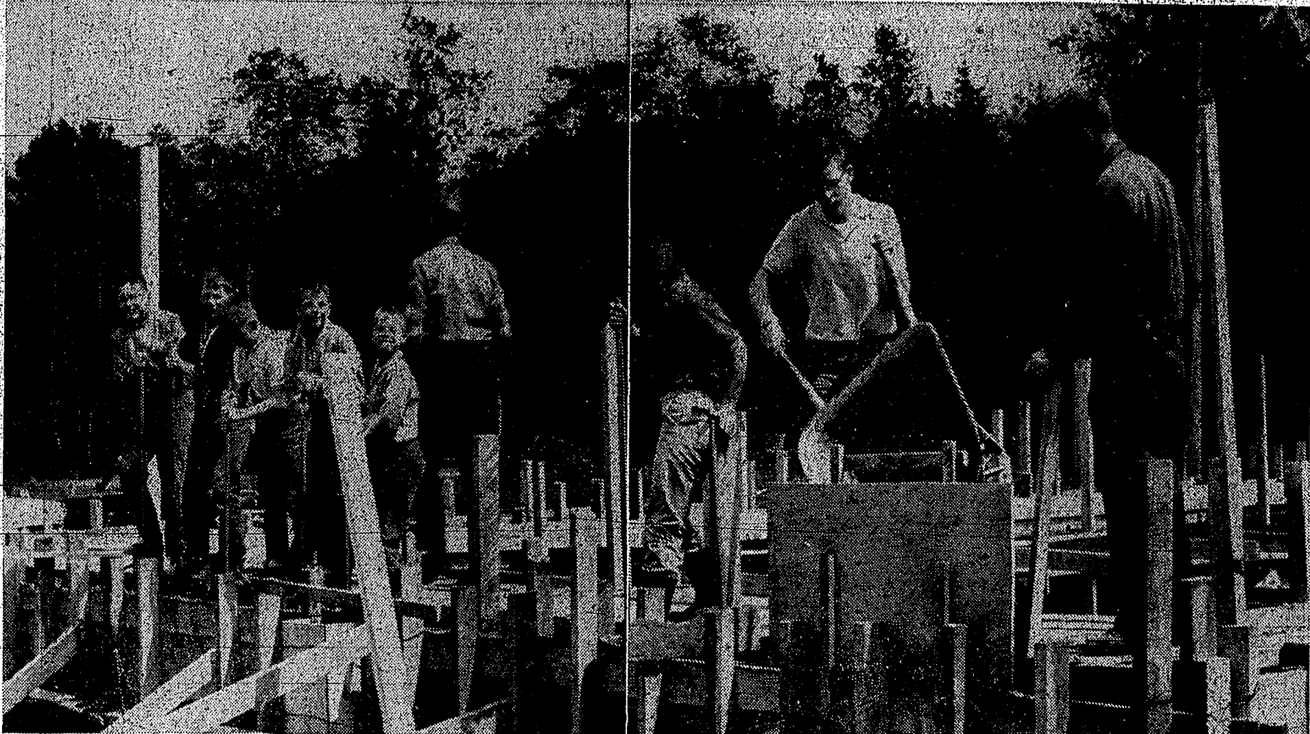
SUNDAY VOLUNTEERS buildings concrete wall of swimming pool seem to be hopelessly blocked by forest of upright boards and two-by-fours but the plank runways are laid out along the top inside. Overseeing the pour from Bob Brown's barrow is
