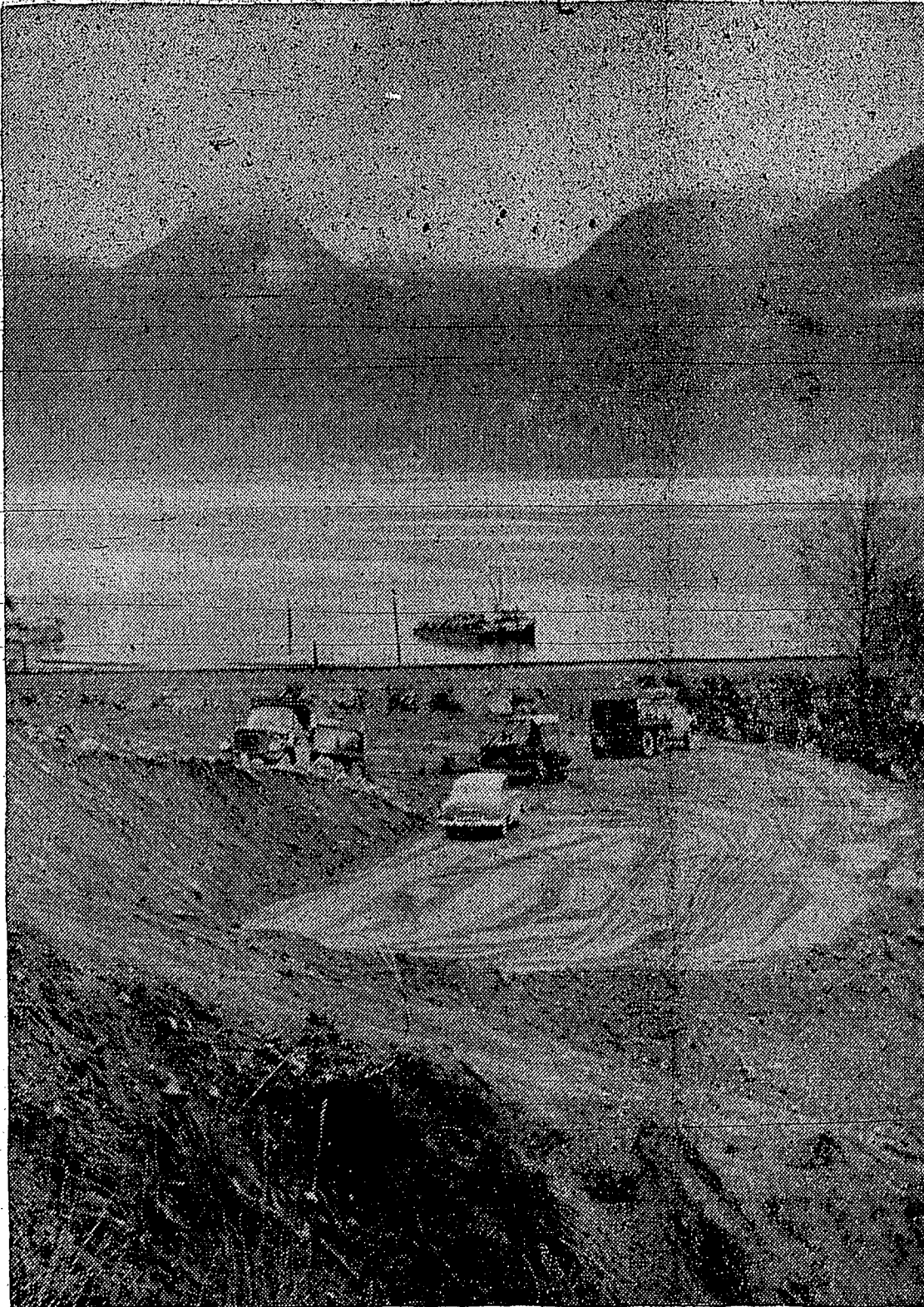
MONTHS OF HAULING is gradually bringing gravel fill at Darrell Bay ferry terminal up to level of PGE tracks and lessening grade to highway from which picture was taken. Wood-fibre, which the ferry will serve, can be seen top center, across the sound. Opening of the extensively renovated pulp mill there is scheduled for April 1. Fill on the other side of the track leading to the yet to be constructed wharf will start soon.
