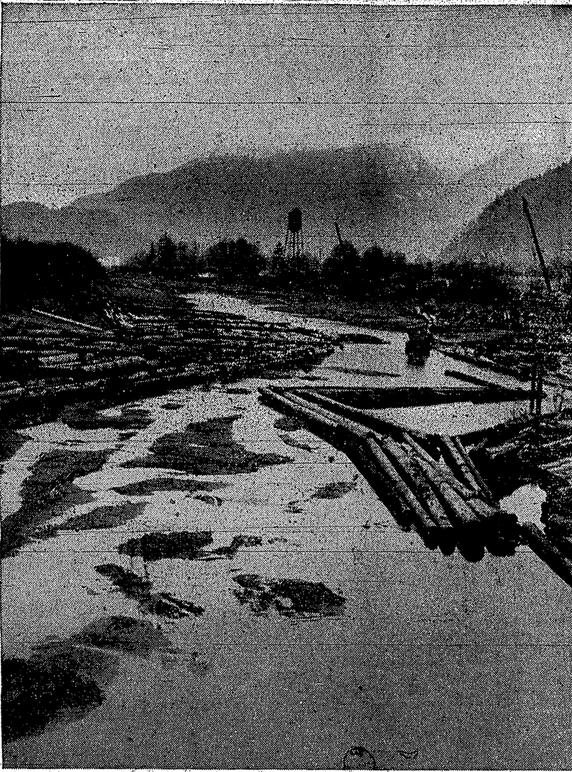
DREDGING of this channel is under way to facilitate movement of log and job is slated for completion in two weeks ago. Dredge started work May, and width of 100 feet is the plan.
